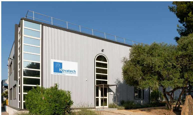
Office, production and warehouse in La Ciotat, south of France
